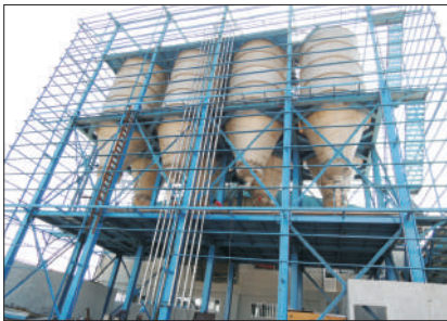
Flour Silo Turnkey Project
