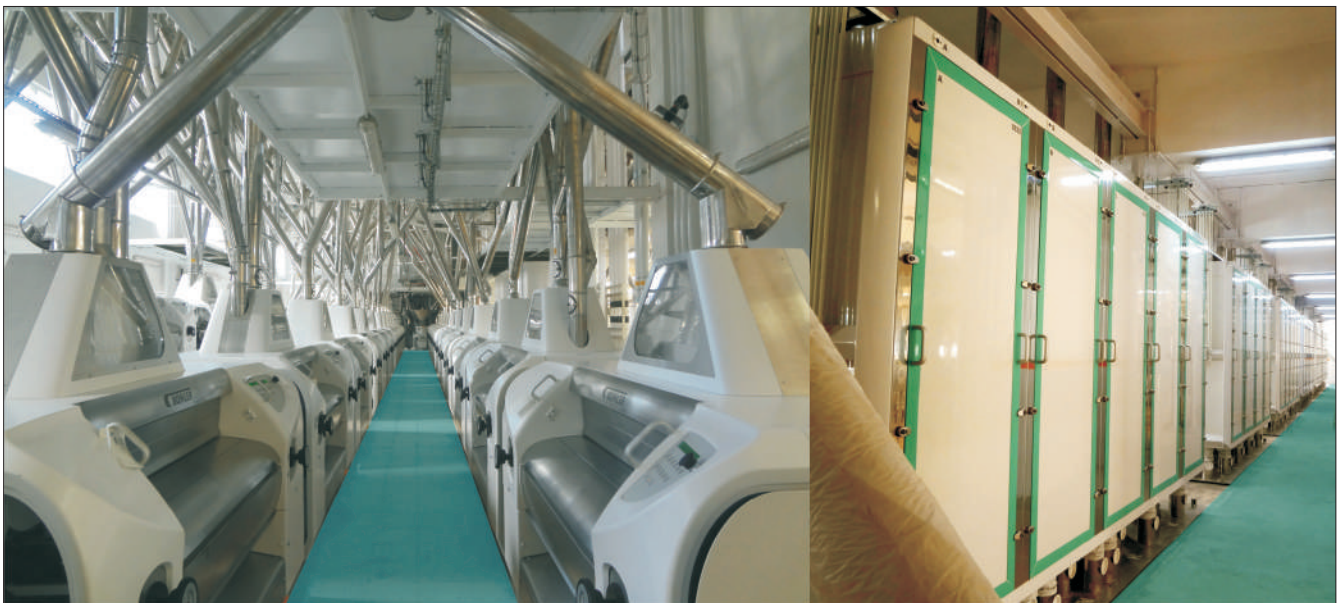
Flour Mills Erection Turnkey Project
